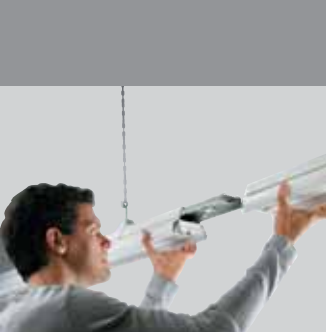
Mechanical connection of the trunking sections by pushing them together.
